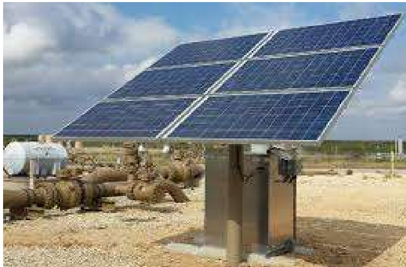
Fig : Cathodic protection of oil pipe lines using PV system .
